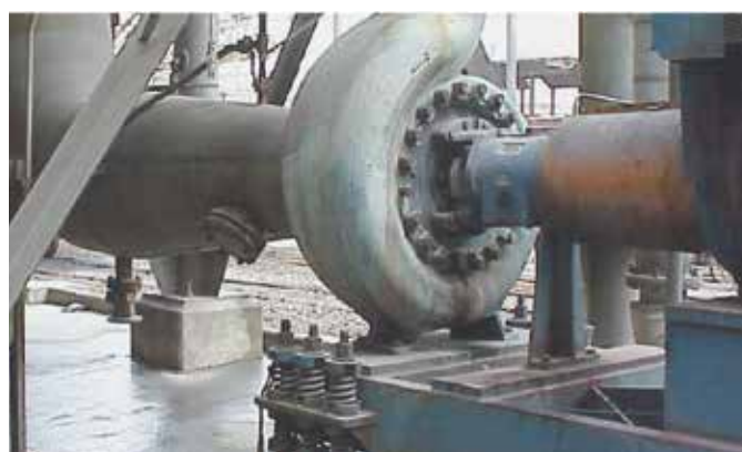
Model 3180XL on difficult high temperature service. Spring-mounted baseplate provided to compensate for thermal expansion.
