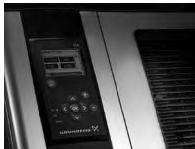
Fig. 22 Grundfos CUE control panel
