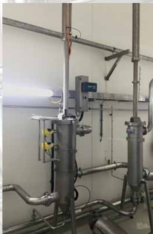
2 pcs. Auto-line® XLE for filtration of brine from brine bath in hard cheese production facility
