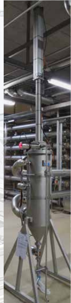
Auto-line XXLE police filter for condensate filtration before UF/RO installation
