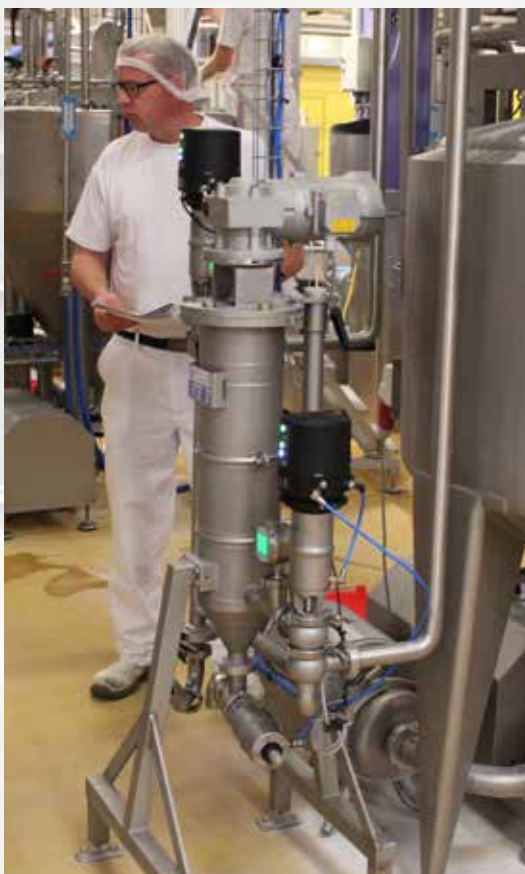
Auto-line® MLR-E for filtration of melt cheese
