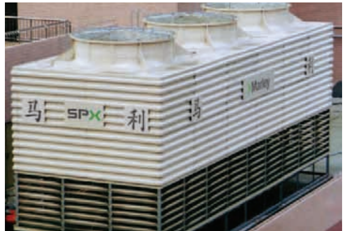
Marley SRC Cooling Tower —Induced draft, counterflow design. Fiberglass field-erected structure. Stainless steel substructure option. Not available in the US, Canada or Europe.
