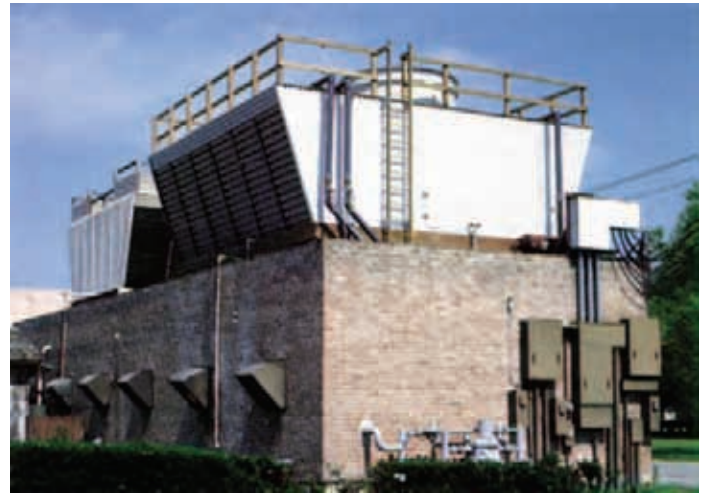
Marley Series 10/15 Cooling Tower —Splash-fill design for use at high temperature or where poor water quality prevents the use of film fill. Wood structure available in treated Douglas Fir or redwood. Tower cells available from 215 to 4,800 GPM.
