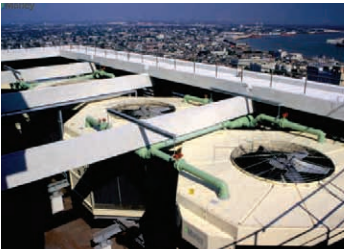
Marley QuadraFlow® Cooling Tower —The first in the industry protected by a five-year total product warranty covering virtually every part of the tower. These fiberglass and stainless steel towers are field assembled to facilitate siting, and are available from 129 to 1,047 tons per cell. CTI Certified.
