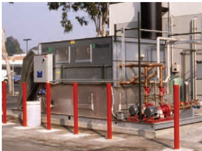
Recold JC Evaporative Condenser —Forced-draft, low profile design. G-235 galvanized steel factory assembled structure. Also available in 300 series stainless steel. Proven copper coil technology.
