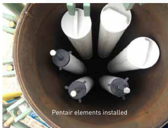
Pentair risers and cores installed
